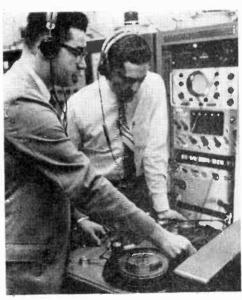
Bell Telephone Lab scientists listen to a tape recording of synthesized speech which was produced by a programmed digital computer.
